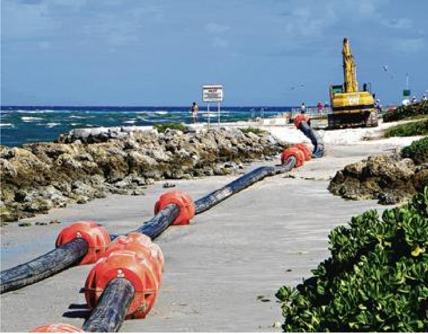
A 2016 dredging project in Palm Beach, Florida, brings 70,000 cubic yards of sand from the bottom of the ocean to the shore.
